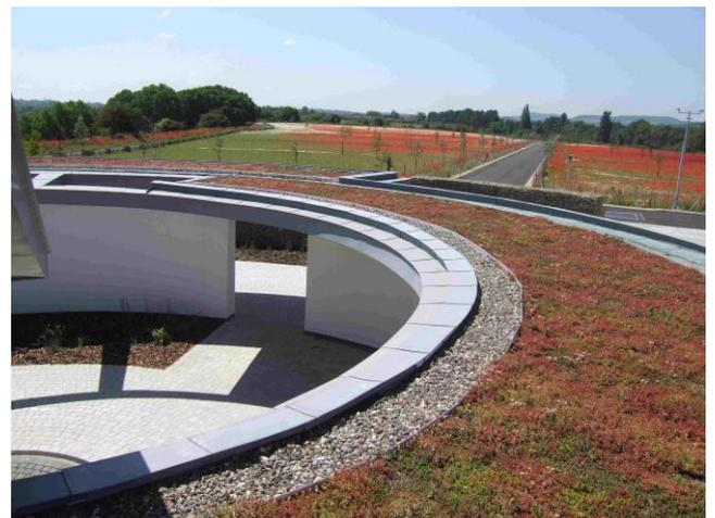
Extensive living roofs are not usually trafficked but are intended to be visual or ecological features. Typically, they have thin substrate layers to minimise depth and weight and are designed to be low maintenance with slow growing vegetation. They are often created to provide habitat for flora or fauna and to enhance building performance by reducing rainwater flow rates and increasing thermal efficiency.
