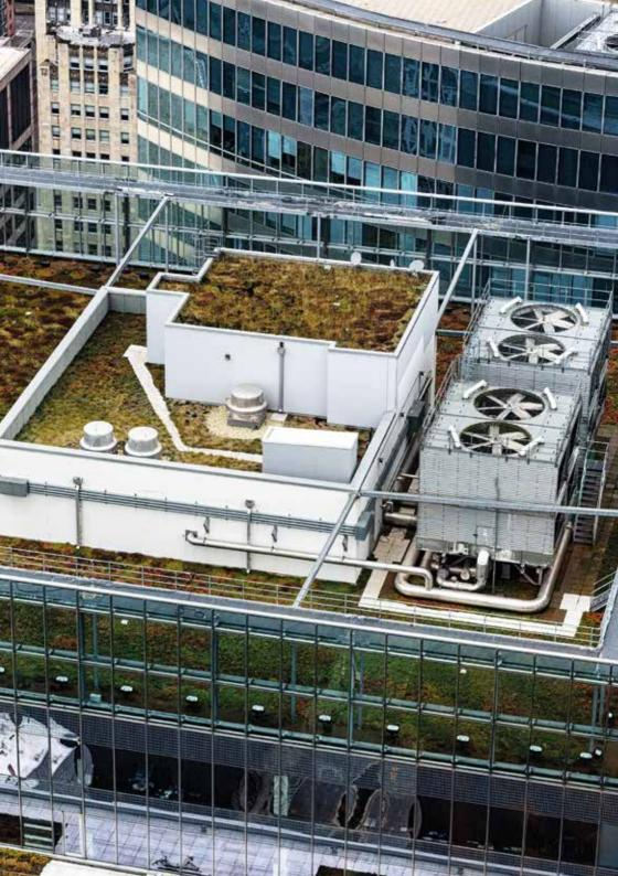
A Blue Roof can be created at either roof or podium level above the waterproofing membrane in a warm roof application and above the water flow reducing layer (WFRL) in an inverted application, and should attenuate water for no more than a 24 hour period from the end of the maximum designed rainfall event. The discharge rate should be calculated to allow the roof to be half empty of attenuated water in a 12 hour period.
