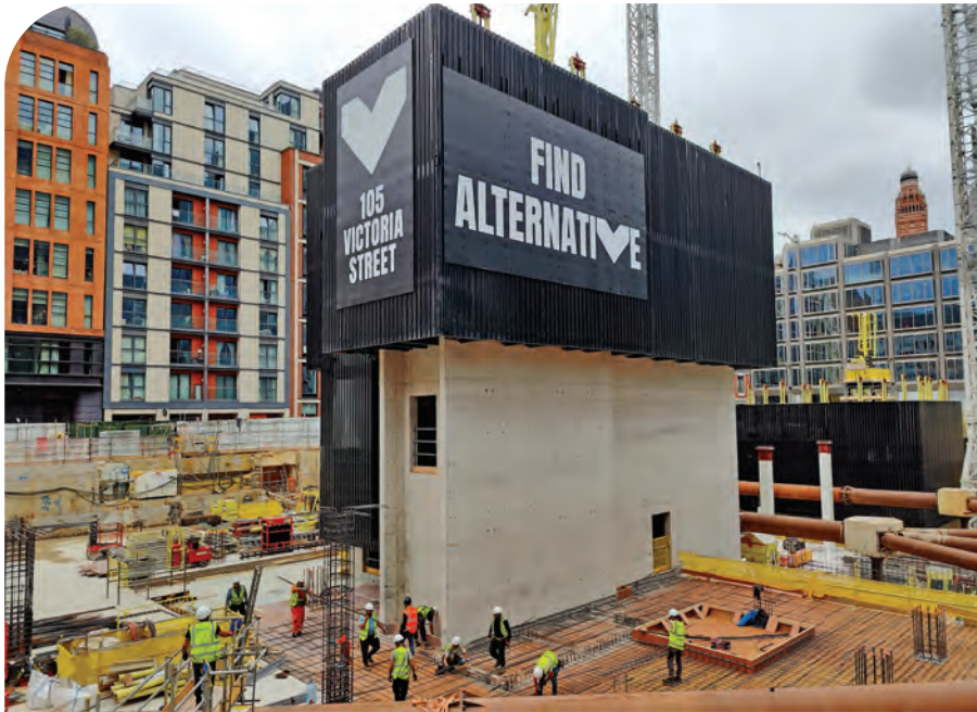
LEFT: Jumpform construction of the core.
