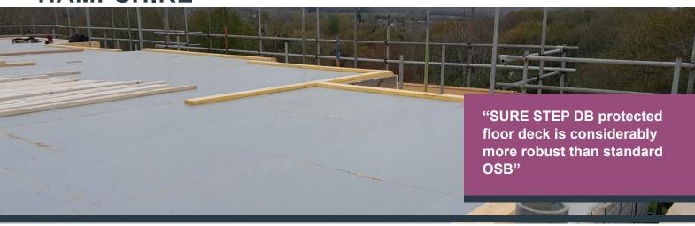
In the village of Sarisbury Green in Hampshire, a new residential development is being built by local developer Alpine Homes Limited, using a closed timber-frame panel system developed by low carbon structures manufacturer VerdeGO Timber Frames Ltd, and part of the build features none other than SMARTPLY SURE STEP DB.
