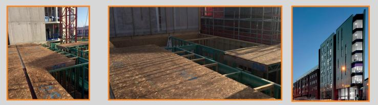
SMARTPLY FR/FR BUILD OSB3 from MEDITE SMARTPLY has been used as a flame retardant flooring solution within a seven-storey, timber frame accommodation building for students of John Moores University and University of Liverpool.
