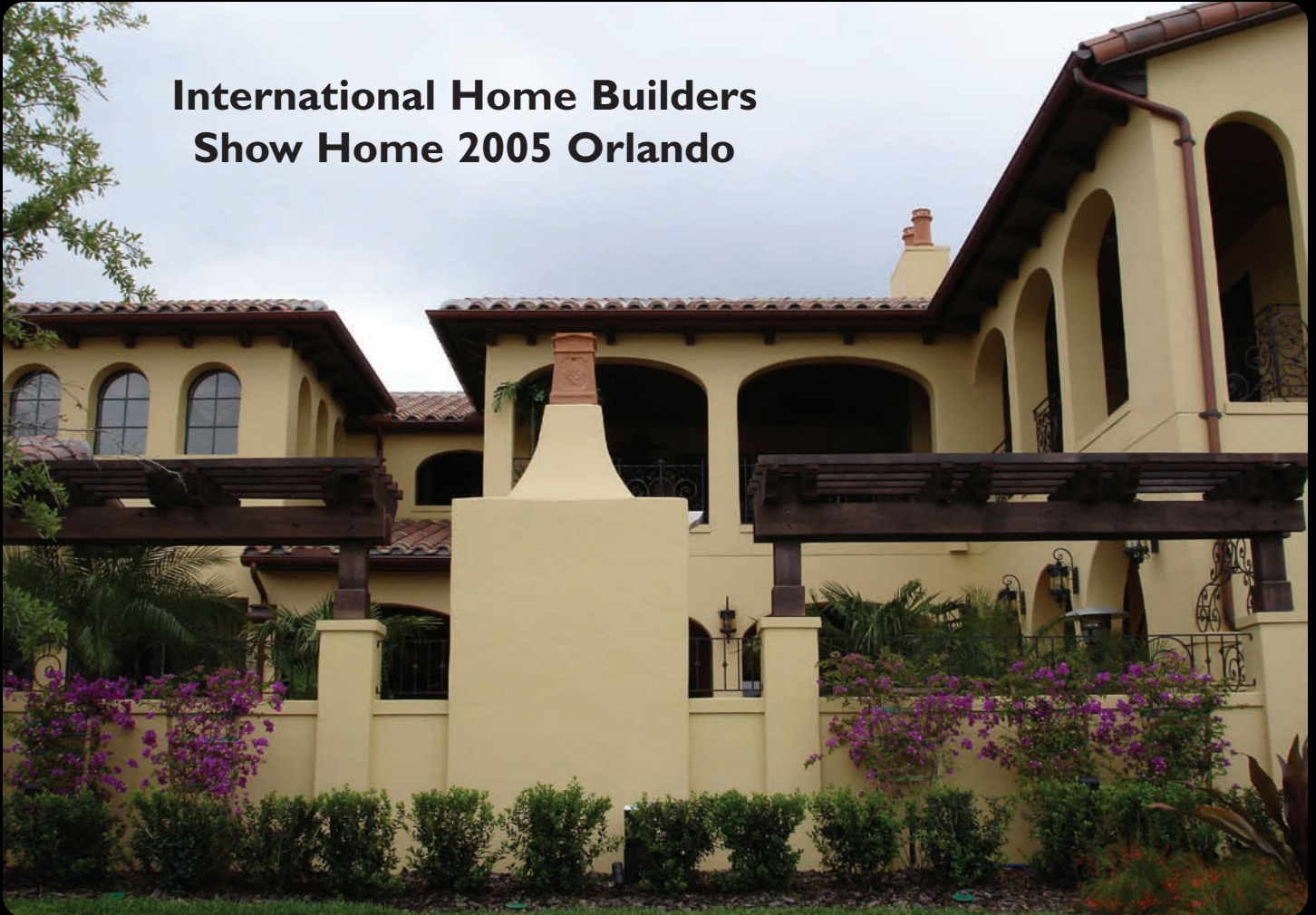
Gutter system 7" half round 20 oz copper gutter with scroll hangers. 4" copper pipe with cast copper clover pipe straps and leaderhead LH014.
