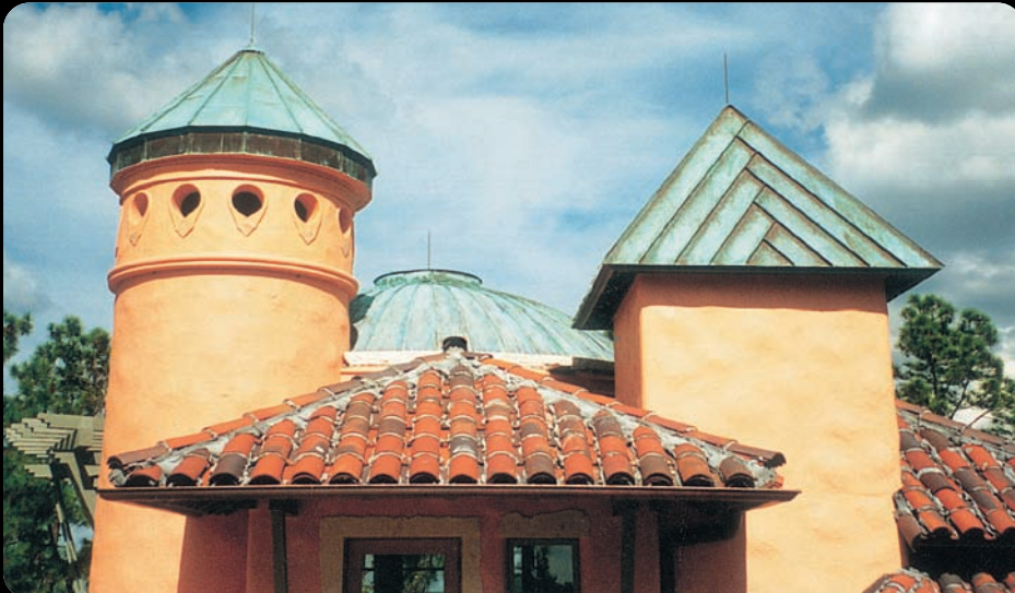
Patina standing copper seam roofs with 6" half round copper gutter
