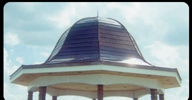
Bermuda style copper panels on gazebo roof
