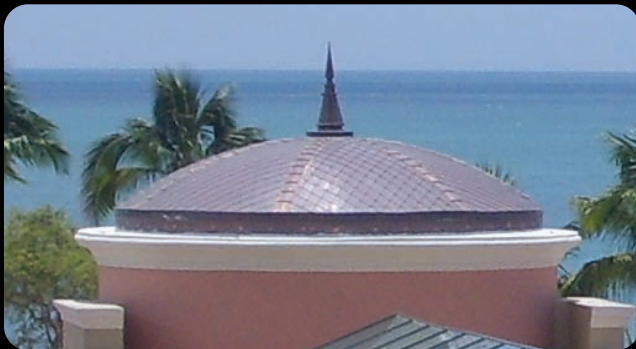
Custom dome fabricated in Antigua covered with copper diamond-shaped tiles as shown below
