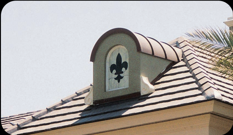
Copper standing seam dormer window
