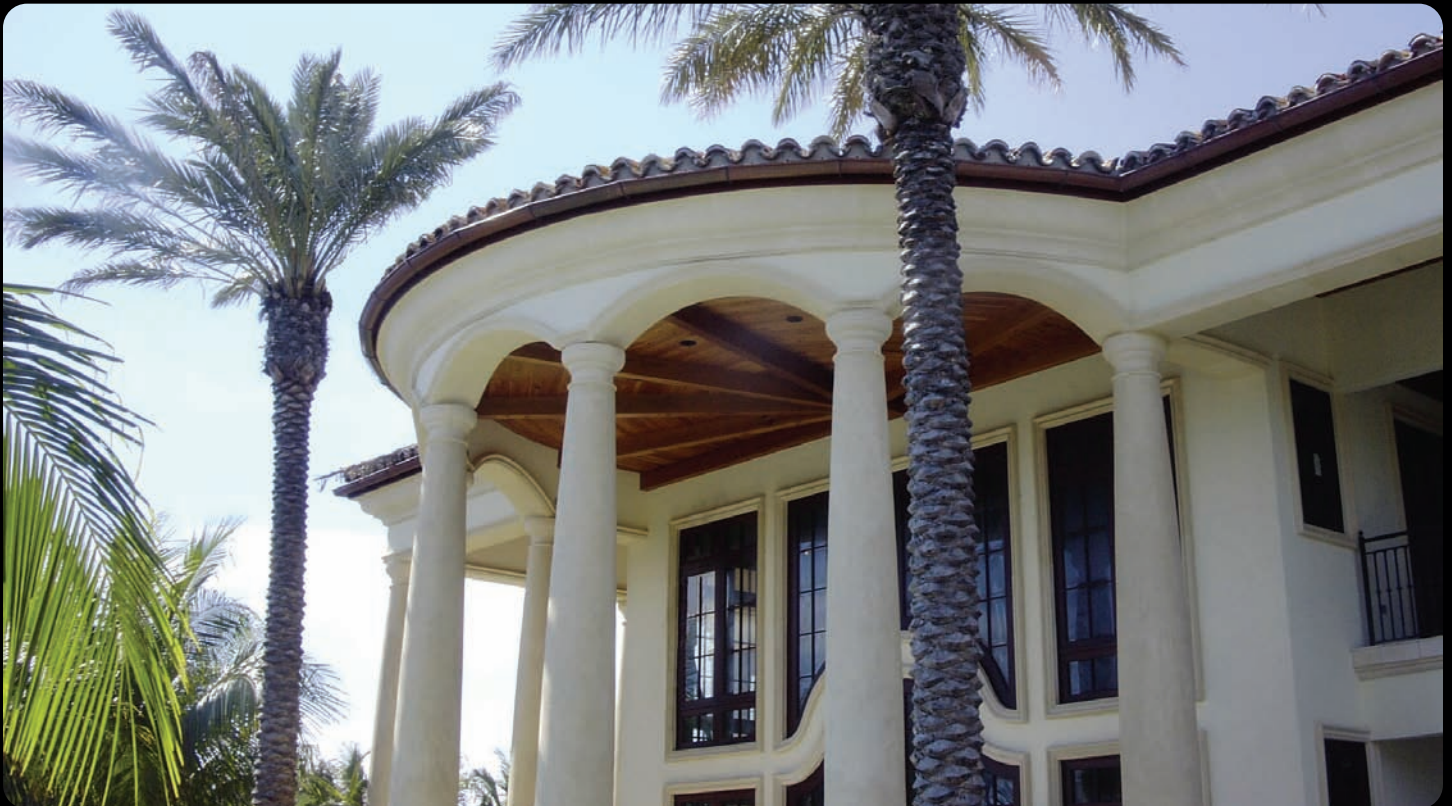
7" half round radius copper gutter installed with scroll hangers.
