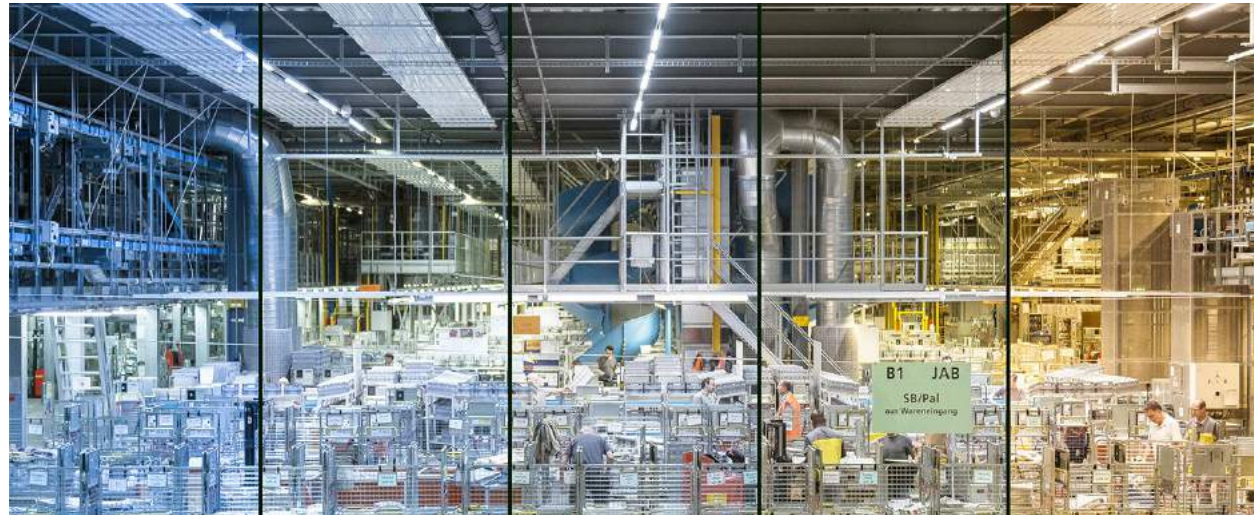
Picture: Distribution centre in Härkingen, conversion from fluorescent lamps to LED, infrastructure (suspension, mounting rails, wiring) of the system remained intact.
